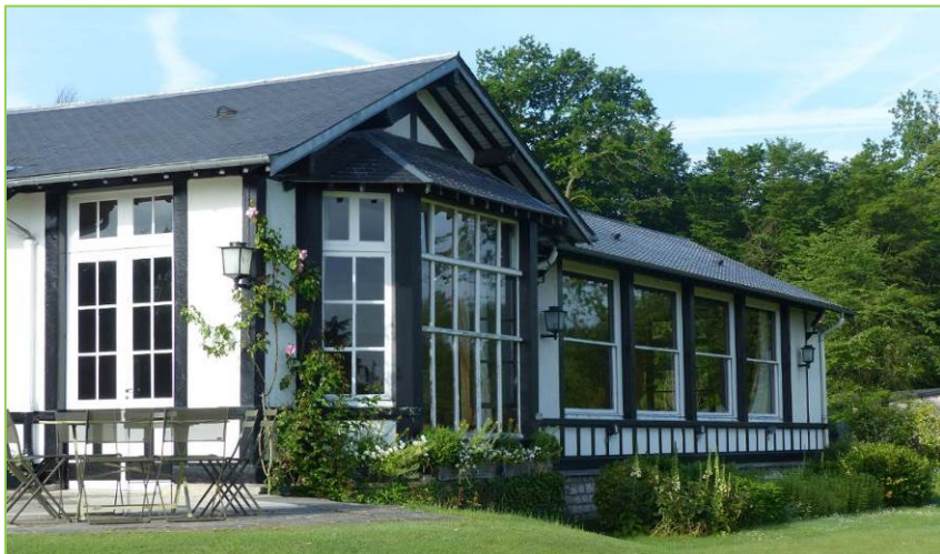
Figure 64 – Le clubhouse © O. Roquinarç'h, 2017.
